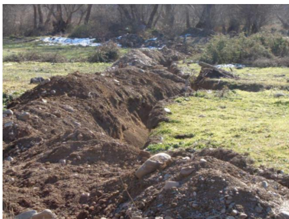
Figure 4.1.3. Trench excavated near Razdara village
